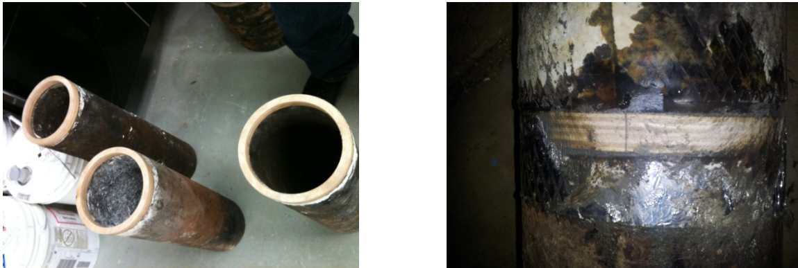
Figure 3: Location of wooden spacer (left) and wooden spacer in between the host-pipe sections (left)
