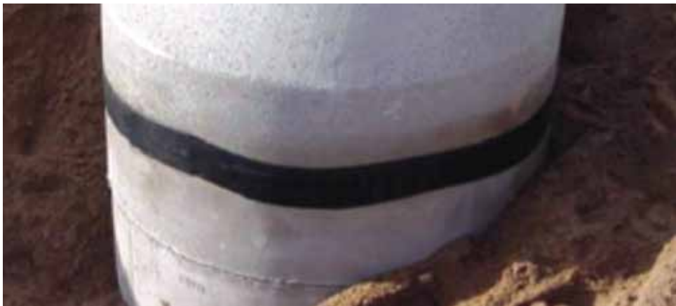
Aquawrap installed around a MH joint
