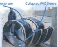
Step 2: Sleeve is jacked into position until it snaps shut & is compressed to the Host Pipe
