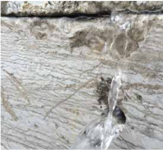
Leaking MH
