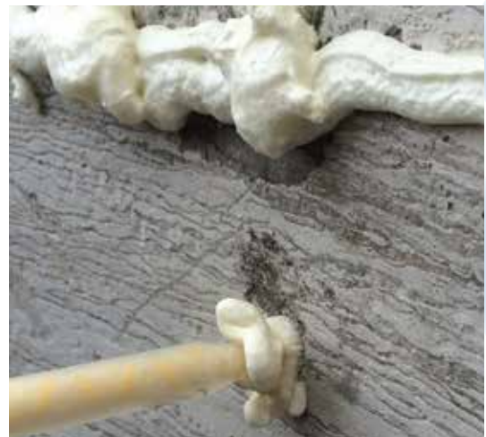
Aquaseal being applied to permanently stop & seal leak
